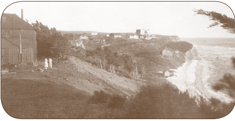
Structure at left probably the big red house, from "Images of America, Moss Beach," by June Morrall
